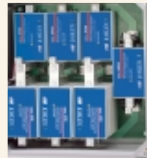
Split-phase 200kA per phase MOV/SAD hybrid
