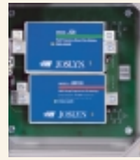
Single-phase 100kA per phase MOV/Filter hybrid
